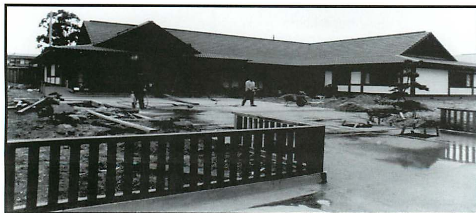
Final Stage of Construction 1976
